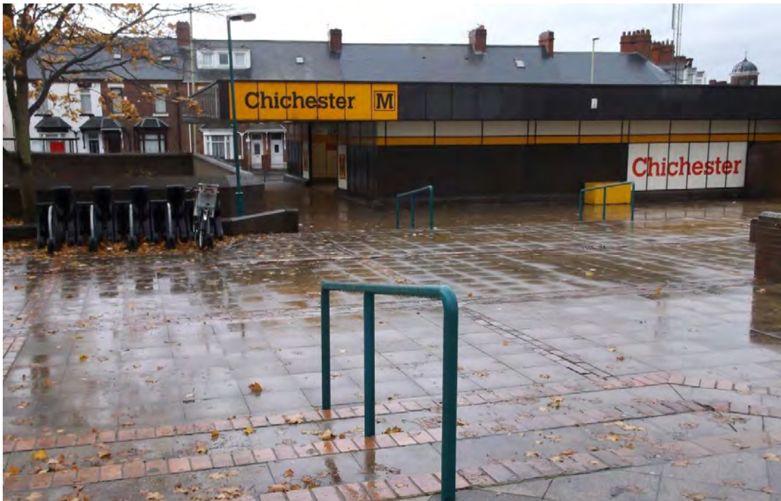
Figure 3.7 – Chichester Metro Station Access with Handrails and Cycle Parking Facilities
